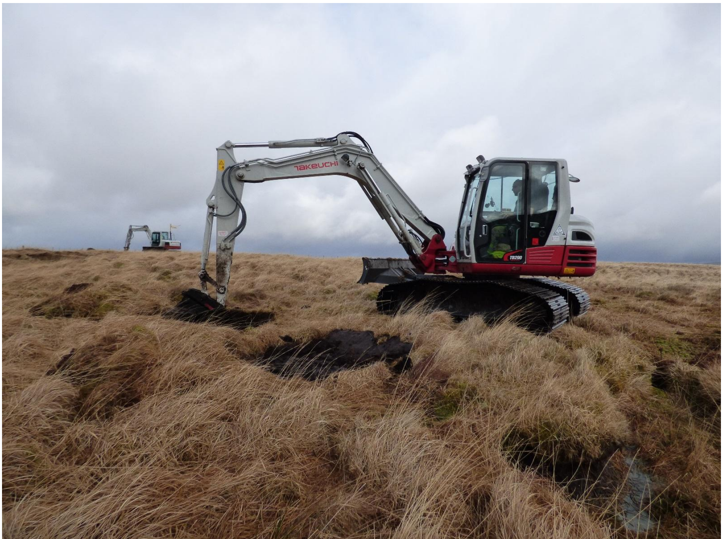
Low ground pressure excavators re-wetting blanket bog at Airds Moss by installing peat dams in ditches © CEI 2015
