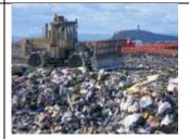
Landfill sites have progressively been improved; operational landfills are lined where appropriate to prevent the leaching of pollutants, and many of them capture the methane emitted from the landfill for power generation or heating.
